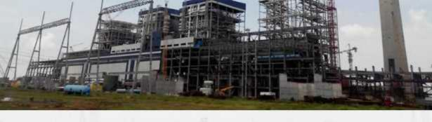
Pre assembly of fabrication structural steel & placement & erection completion of alignment, welding including bolting of TG Unit 2, 3, mill & bunker.
